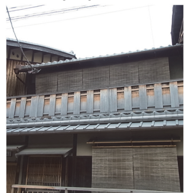
Figure 15. The facade of ho8 having a handrail colored in light brown
